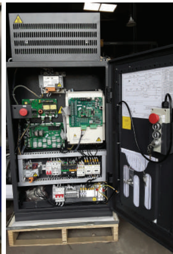
INTEGRATED CONTROL CABINET-NICE 3000
